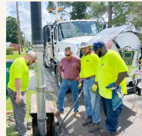
The city had a vacuum truck contractor checking out problem culverts in July to make sure those culverts are clear as part of its pro-active hurricane season preparations.
